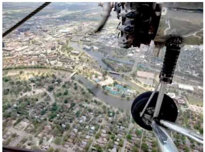
Directly in front of the wheel is Wichita's Keeper of The Plains statue and Exploration Place, both in view of the Arkansas River.
