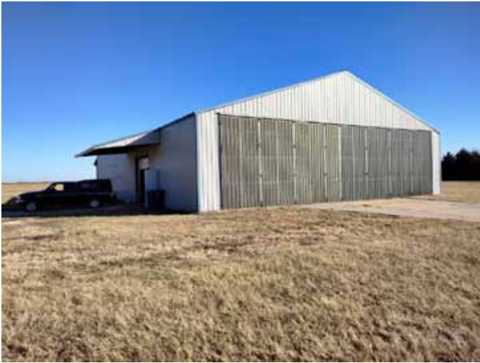
Hangar faces west, short taxi to the grass runway. Airpark is 18 miles from my home.
