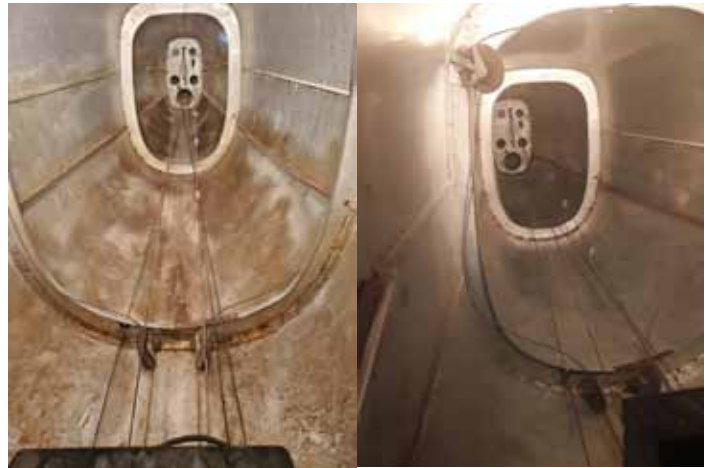
Cleaning on the 120, before & after.
